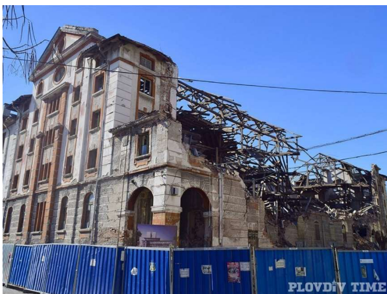
Figure 15 A tobacco warehouse that was deliberately set on fire in order to build new residential buildings on its site in Plovdiv (plovdivtime.bg 2022)
