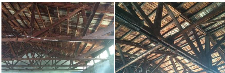
Figure 14 Roof construction of a building next to Montana Airport, Personal archive. (Петров 2016)
